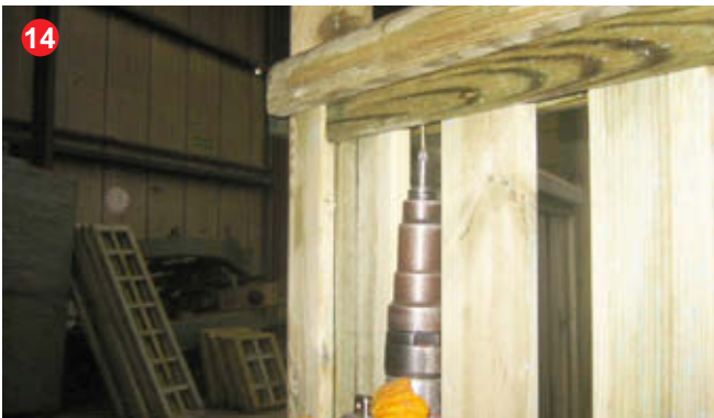
14 Secure hand rails by screwing through fence into handrail using 3 x 40mm screws.
