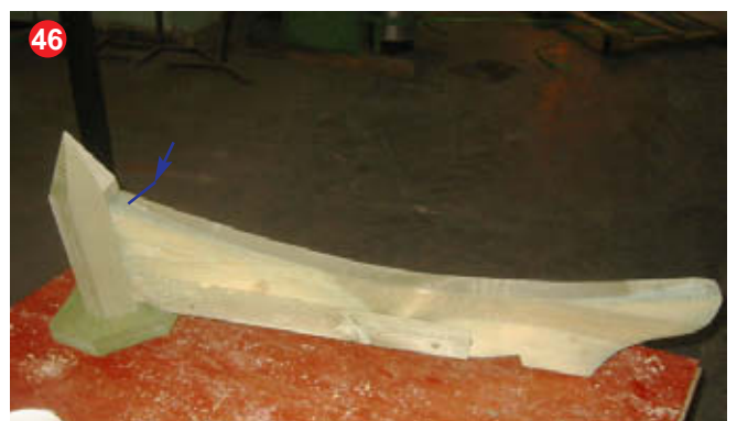
Drill hole and screw top roof bearers to centre finial using 1 x 70mm screws.
