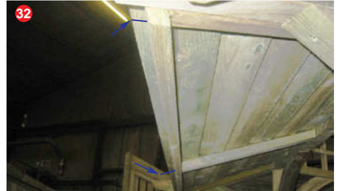
Underneath view of roof coverstrip attachment.
