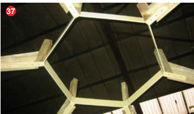
Attach the remaining 2 bearers to the metal ring and to the main assembly as before.
