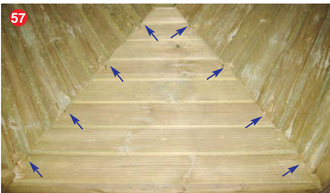
57 Secure each floor panel down using 8 x 50mm screws per panel.
