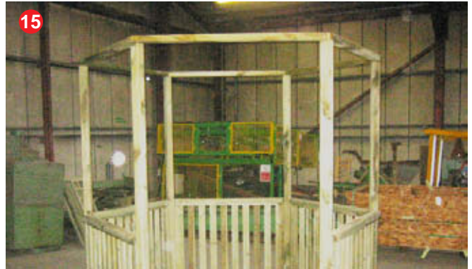
15 Upright top frames are positioned as shown.
