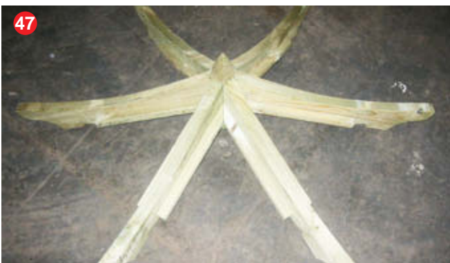
Shows all top roof bearers attached to centre finial.
