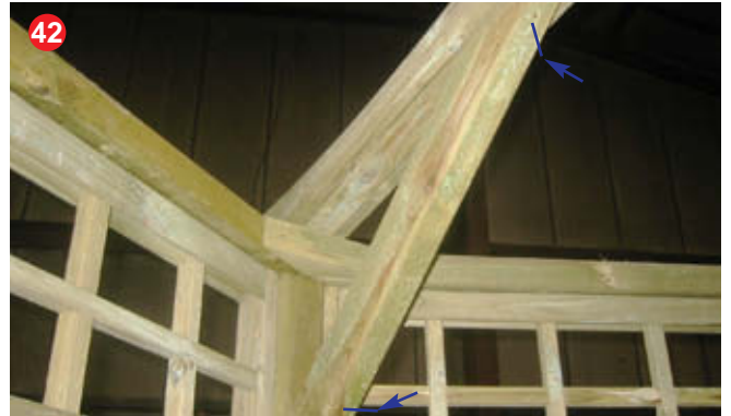
Secure each roof support with 2 x 50mm screws.
