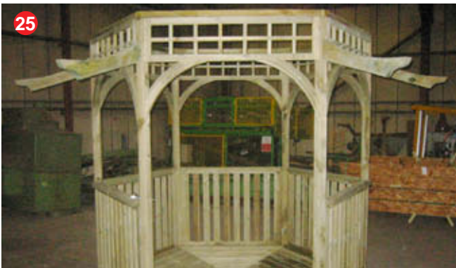
25 Shows Lower roof supports in place.
