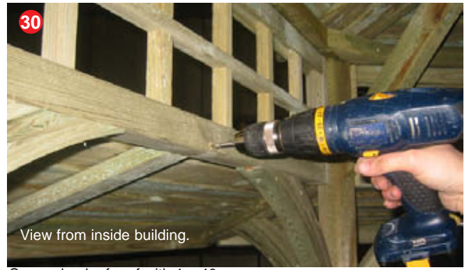
Secure back of roof with 1 x 40mm screw.
