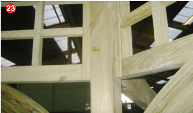
23 Secure the lower roof bearer using 1 x 130mm screw per upright.
